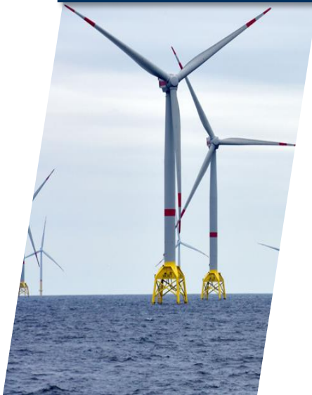
Offshore Wind Farm
